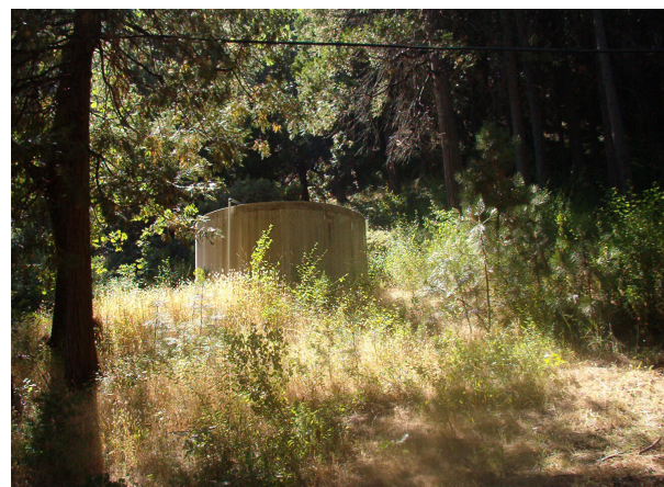
CDF fire suppression water tank
