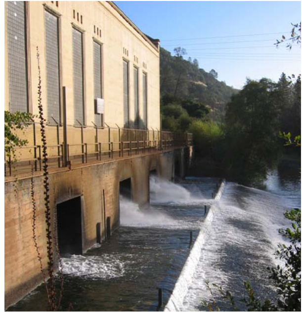
Electra Powerhouse discharge
